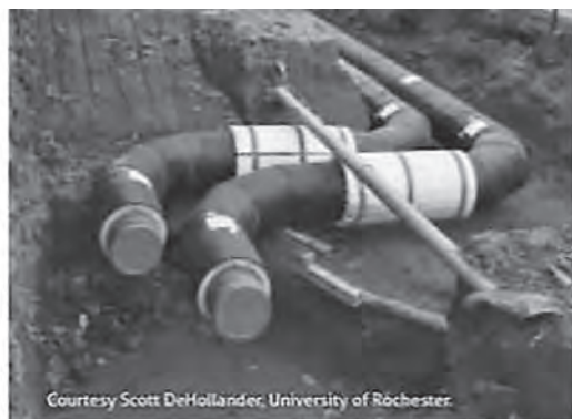
Thin-wall EN253 pipe installation at the University of Rochester in 2017.
